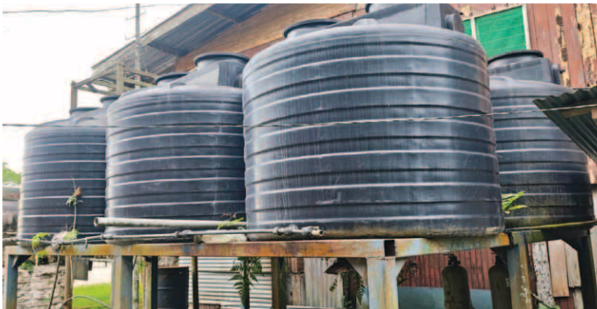
Improving rainwater harvesting system by addition of 6 tank each 1,500 Litre in site facility.
